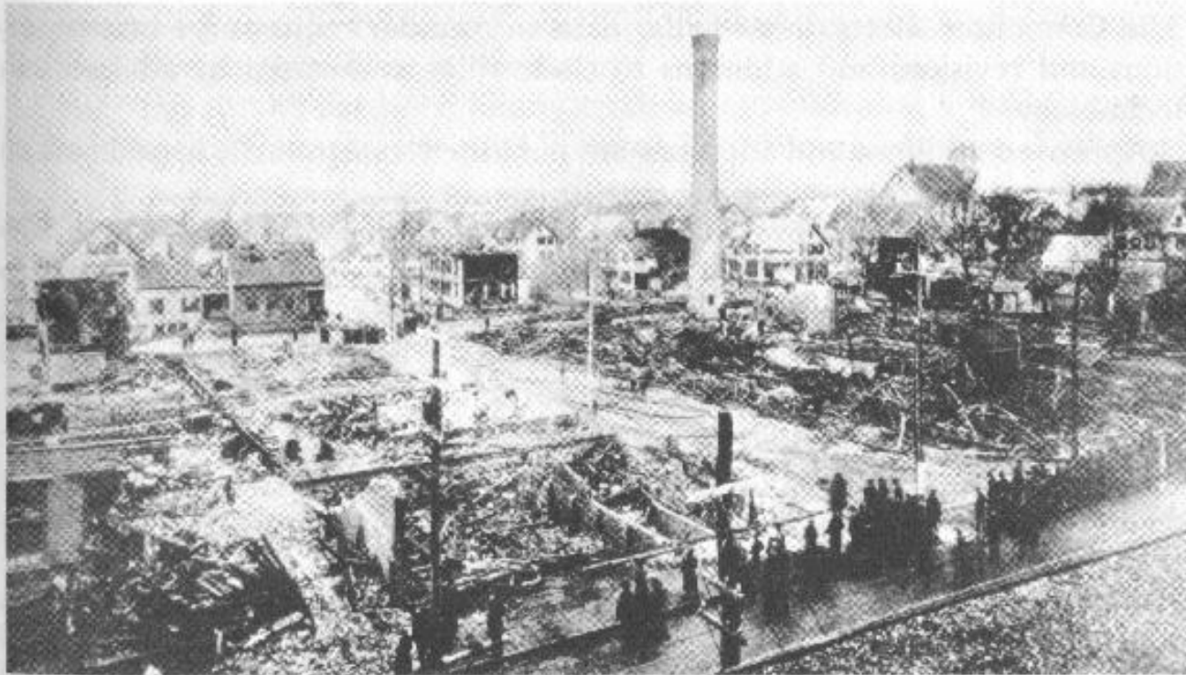
Fig. 1.2 Shoe factory after the boiler explosion of March 20, 1905 which led to the adoption of many state boiler codes and the ASME Boiler and Pressure Vessel Code . (Courtesy of Hartford Steam Boiler Inspection & Insurance Company)
